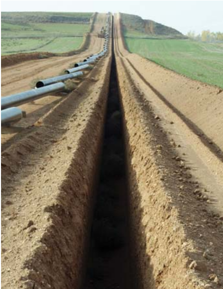
Figure 2: Typical underground pipeline construction
