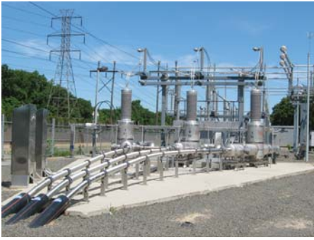
Figure 1: 138 kV AC superconductor power transmission cable operating since April 2008 in Long Island Power Authority's grid.
